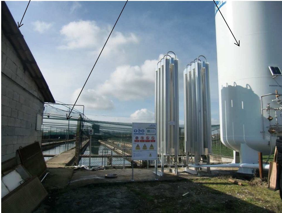
8 building for feed storage, second entrance and silos for oxygen
