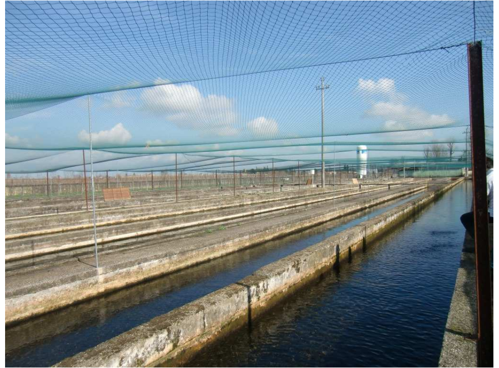
9. Overview of the raceways
